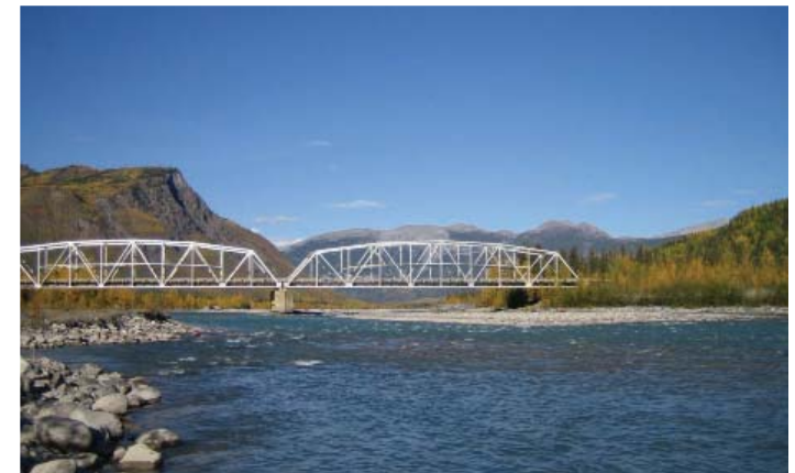
Racing River Bridge photo courtesy of T. Forest
