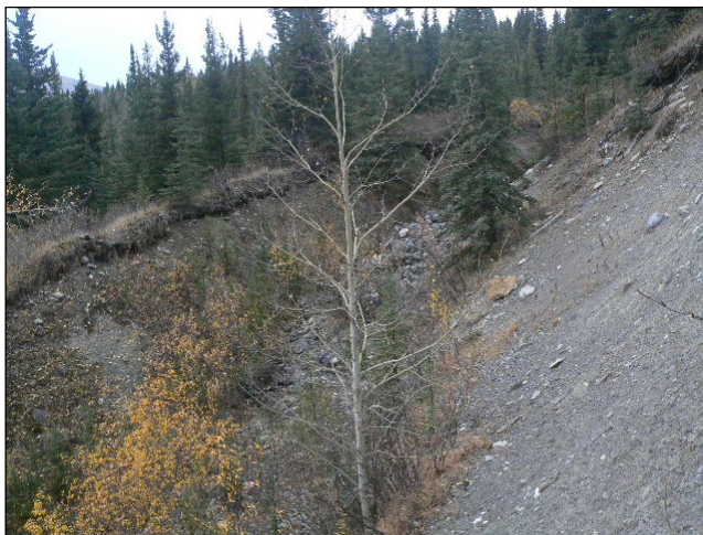
Figure 15: Gully where original road bed is transitioning to an washed out.
