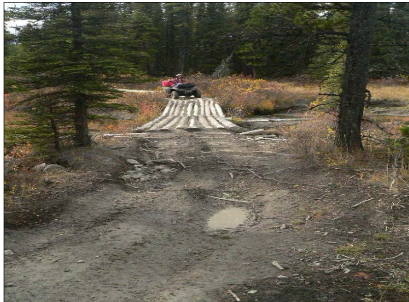
Figure 19: Typical corduroy bridge in Redfern-Keily Provincial Park.
