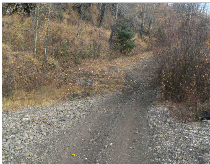
Figure 4. Berm on lower slope position of road restricts water movement.
